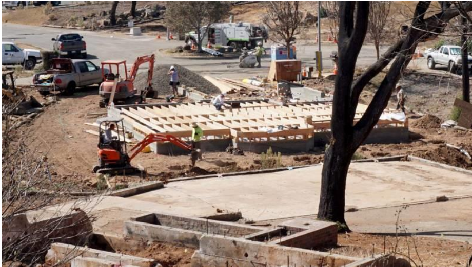
The Tubbs Fire swept away about 5 percent of Santa Rosa's housing stock. (Lauren Sommer/KQED)
