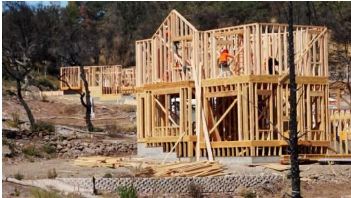
A house burned in the Tubbs fire under construction in Santa Rosa. ( Lauren Sommer/KQED )
